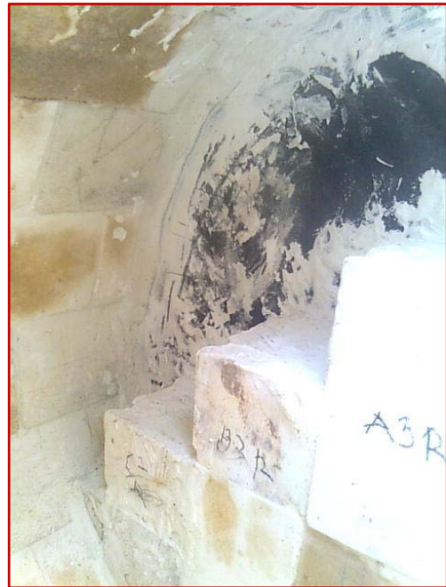
Plate 6: Porcelain liners set in bond material Photo: Oresegun, A.O. fieldwork (2012)
