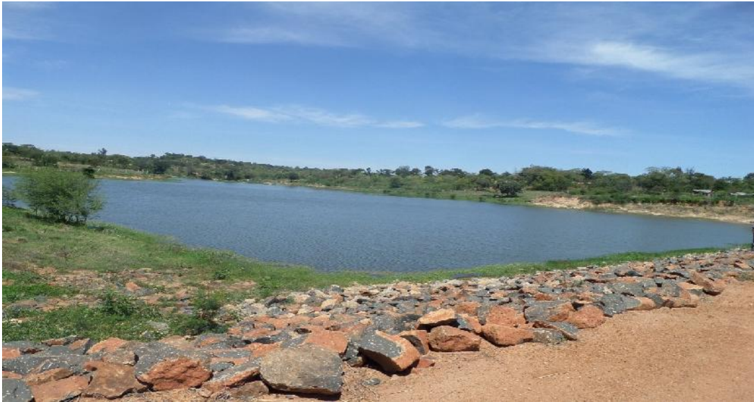
Figure 6: A dam constructed on a seasonal river in Kitui Central
